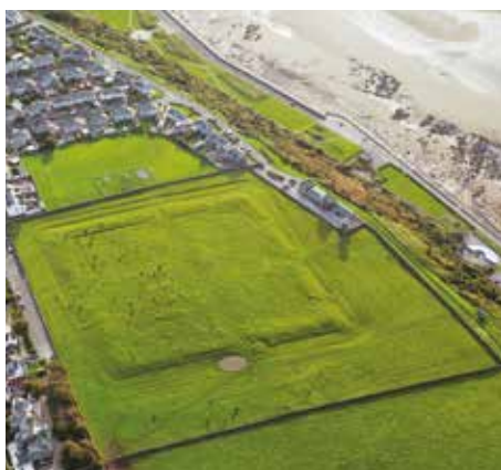
Aerial view of the fort at Maryport.
