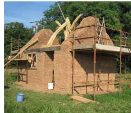
Campfield Marsh clay dabbin under construction
