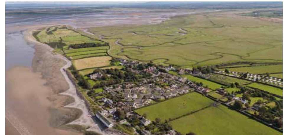
Aerial view of Skinburness looking north
