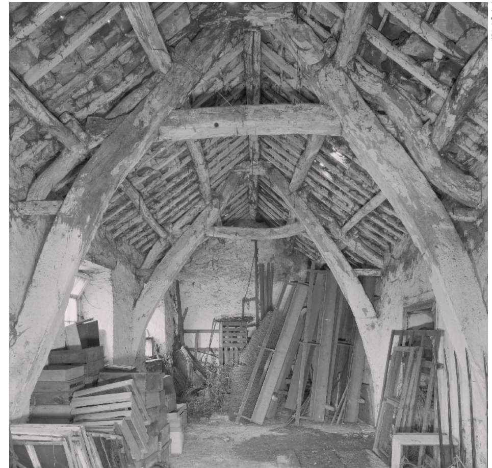
Interior of a cruck barn, Great Orton
